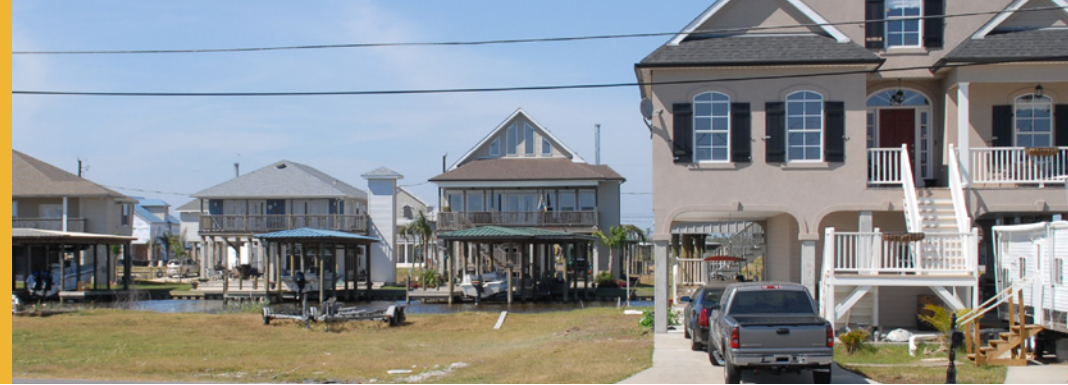
April 4, 2006 — This 100% mitigated community in Empire, Louisiana received no damage from Hurricane Katrina because all homes are built above the flood plain. Marvin Nauman/FEMA
