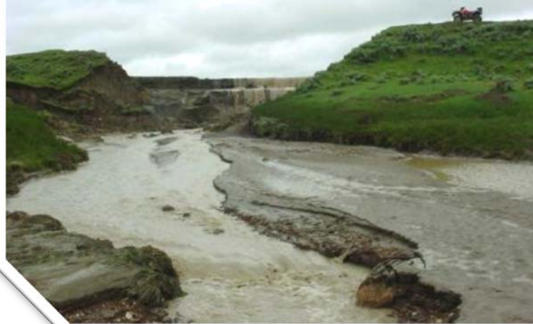
7 Tree dam – Garfield Co, failed May, 2010
