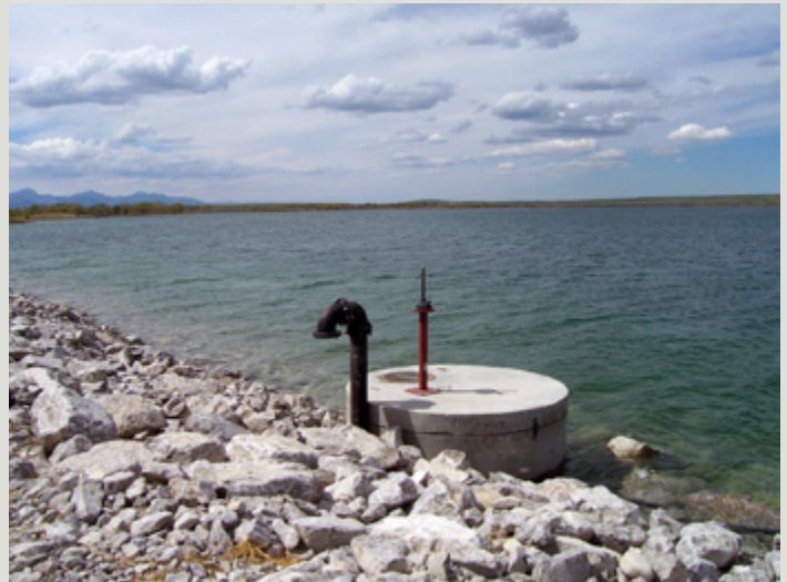
Eureka Dam, Teton County
