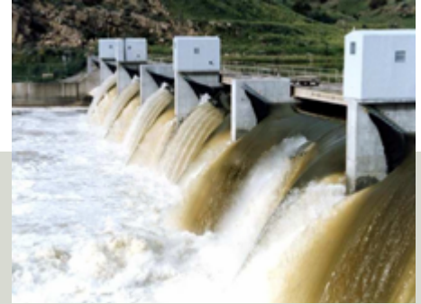
Toston Dam, Broadwater County
