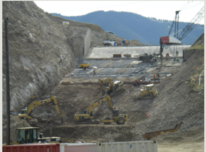
Ruby Dam spillway under construction, Madison County
