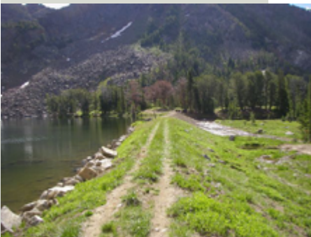
Noble Lake Dam, Madison County
