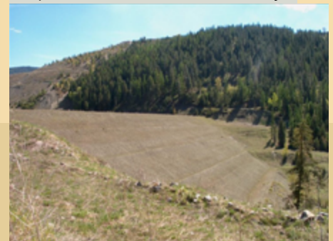
Kootenai Development Impoundment Dam, Lincoln County
