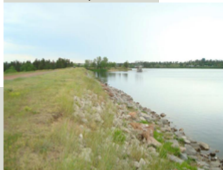
Castle Rock Reservoir Dam, Rosebud County
