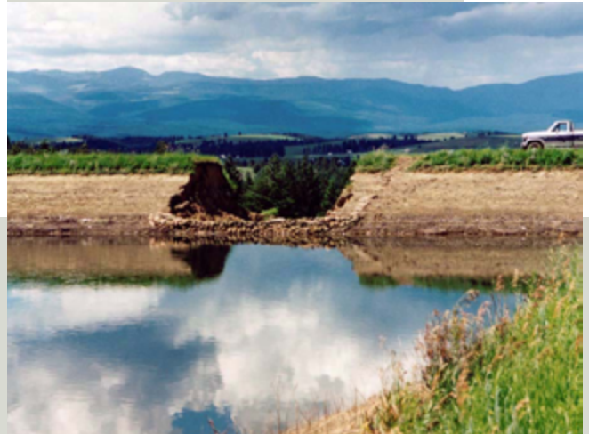
Eureka Wastewater Pond Dam, Lincoln County
