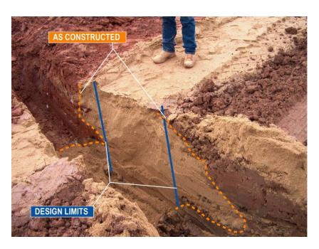
Figure 16 - "Christmas Tree Effect" in Chimney Filter Placement
