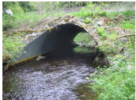
Open bottom arches work well for larger channels, although accommodating spans more than 10 feet becomes challenging.
