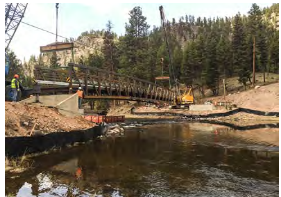
Concrete abutments are generally preferred, and must be protected from scour at the toe. Note the silt fence in place during construction to minimize turbidity.
