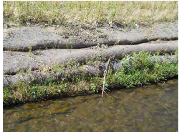
In low erosion/scour locations, toe protection may be “soft” techniques such as coir logs or biodegradable fabric lifts.
