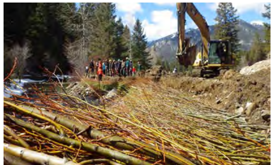
Clean plant material greater than 0.5 inches in diameter is preferred.
