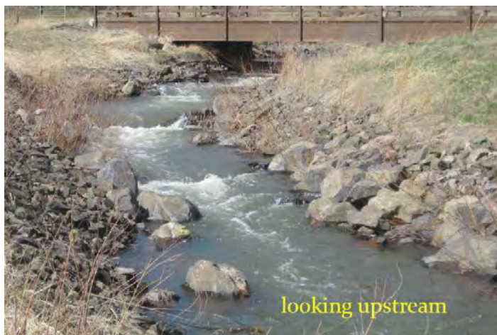
Roughened bypass channel with rock weirs.
