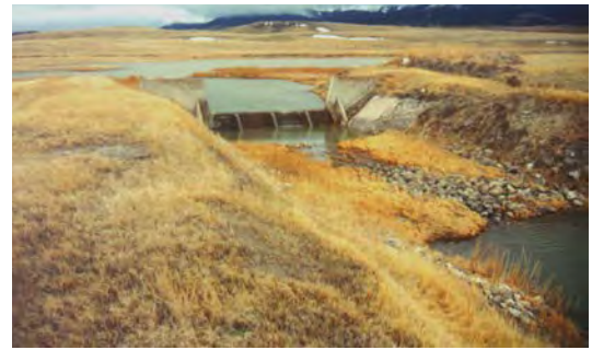
This large concrete structure functions as a Cipoletti type weir.
