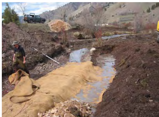
Restoration of channel geometry goes hand-in-hand with revegetation efforts.
