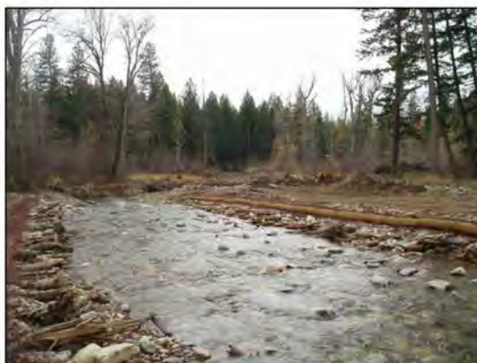
Example of a constructed vegetated soil lift type 1
