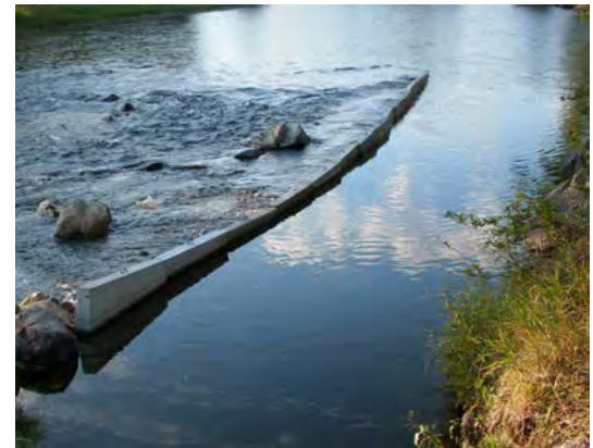
Blocks can reduce the need for streambed disturbance associated with gravel berms. Blocks should be removed following irrigation season.
