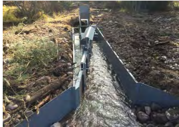
Vertical flat plate screens rely on paddle wheels to power the cleaning brushes. Bypass water returns young fish to the river channel.
