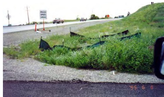
Silt fence helps prevent sediment delivery on newly constructed roads, but does not substitute for proper drainage features.
