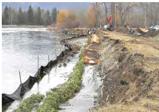
Silt fence can help isolate flowing water and minimize downstream sedimentation.
