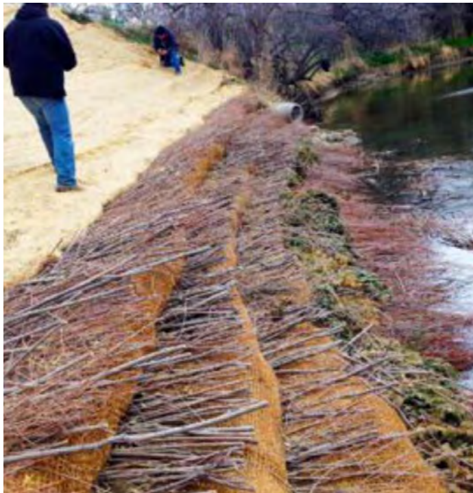
Soil lifts may be constructed with multiple layers. Live brush has the best chance of establishment closest to the water table.
