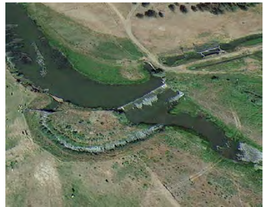
Engineered riffle bypass provides fish passage.
