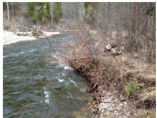
Projects to stabilize eroding streambanks require a 310 permit.
