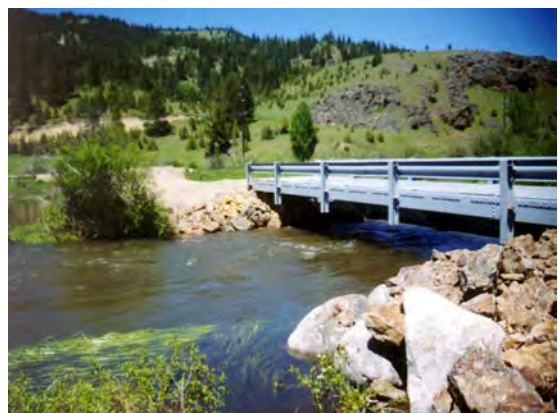
The structural beam on many railcars hangs low and ends up falling below bankfull elevation, which presents risks during high flows.
