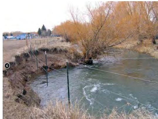
Incised channels typically have bankfull heights below remnant floodplains. Channelization can result in incised channels.
