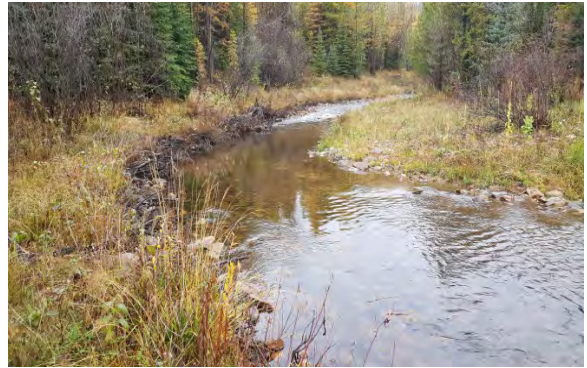
A brush matrix provides short-term stability and roughness. Native sods mats, willow cuttings, and nurse stock are planted to ensure long-term stability.
