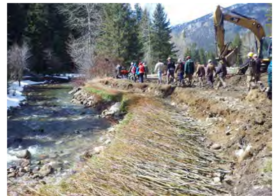
Live brush layers can be used to form a toe where scour depths are not expected to undermine the treatment.
