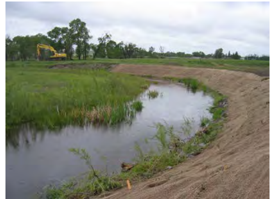
Stream banks are sloped to a 1.5:1 or 2:1 angle and covered with biodegradable geotextile fabric. Toe protection is frequently brush or willow layers. Same location as above photo.
