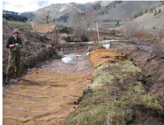
Restoration of streambanks using bioengineering techniques can provide excellent bank stability and promote natural channel function.
