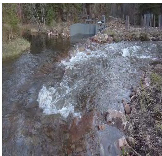
The diversion in the photo above was replaced with a engineered riffle structure, which allows fish passage and maintains natural stream processes.
