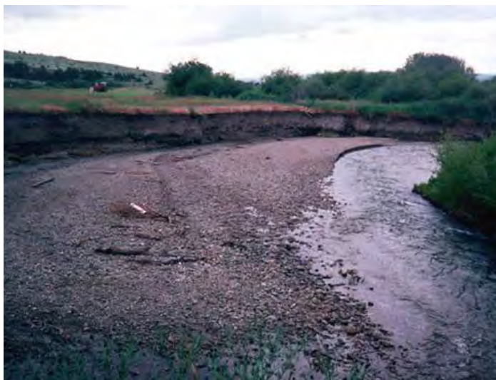
Eroding terrace on Rosgen C3 channel type before restoration.
