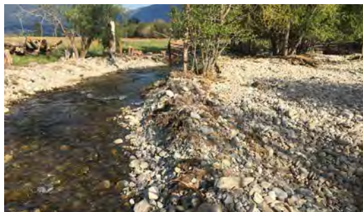
Attempting to control flooding on aggrading channels with excavation and berms is rarely successful because the channel continues to fill.
