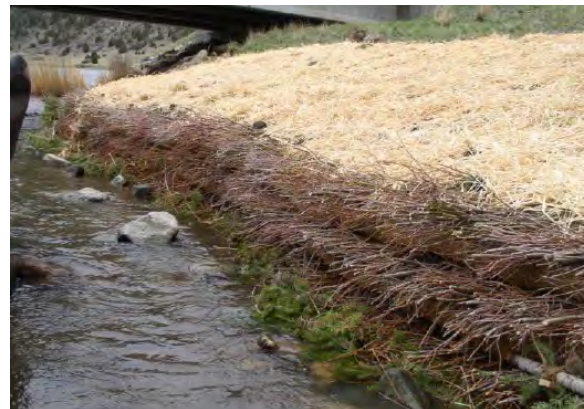
A conifer fascine toe with three soil lifts provide contextually appropriate treatment to stabilize this bank on the Madison River.
