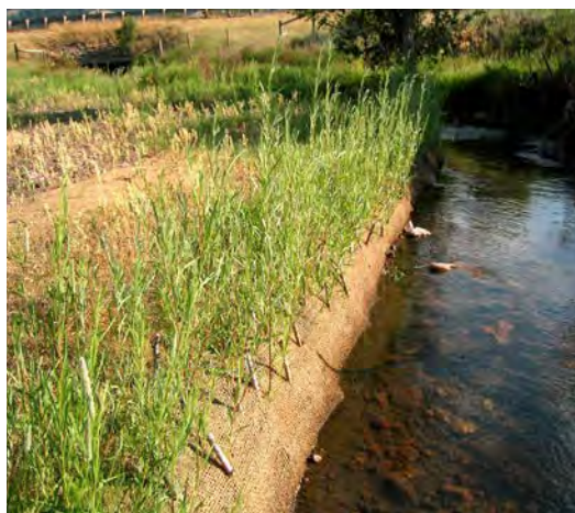
Creating an appropriate moisture regime is key to establishment of wetland and riparian species. Willow cuttings should be placed deep enough to intercept the water table.
