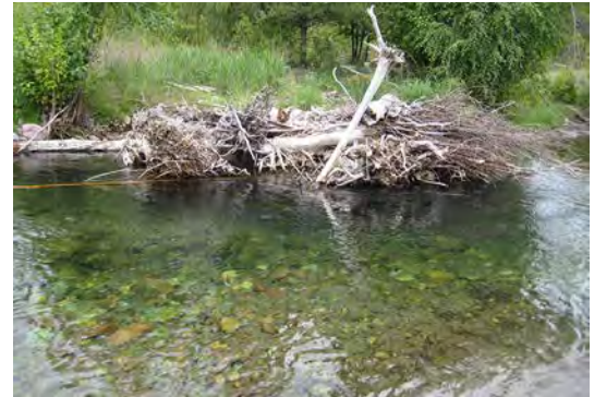
Constructed log jams create hydraulic diversity and can provide bank protection.
