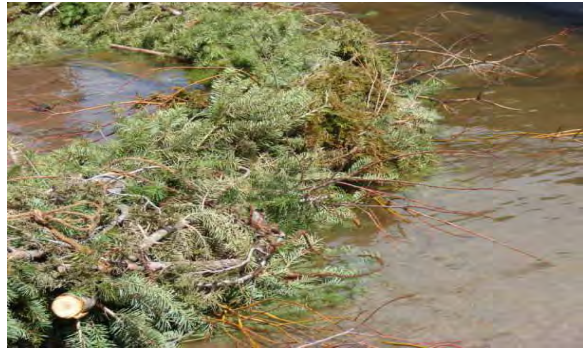
Conifer fascine provides added hydraulic roughness and habitat complexity compared to coir logs or rip-rap
