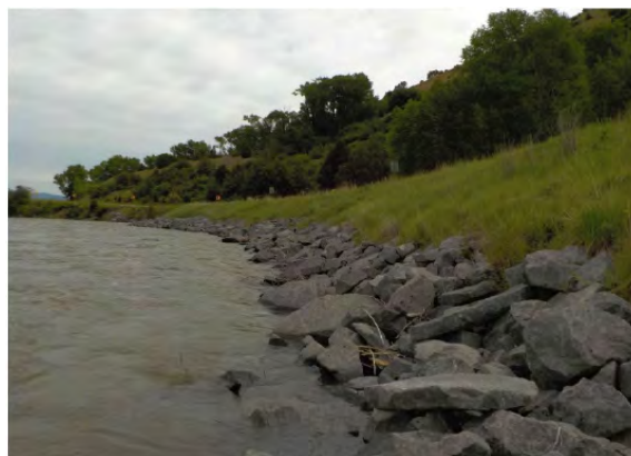
The upper bank stabilized with natural geotextile fabric has been successfully revegetated for aesthetic value. Incorporating willows within the rip-rap can further enhance natural processes.
