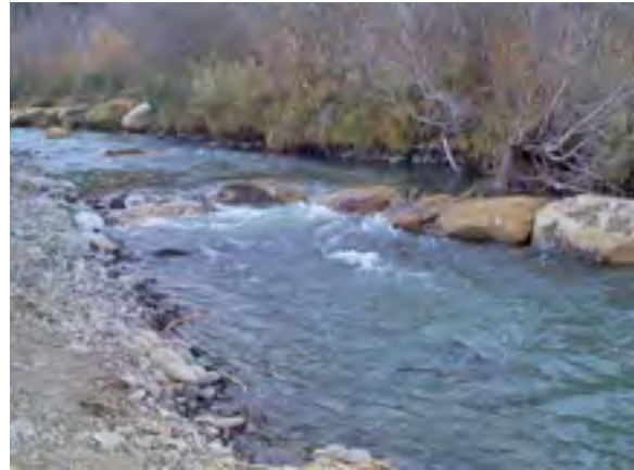
Barbs are constructed with a low sloping profile and gently “roll” the current away from the bank.
