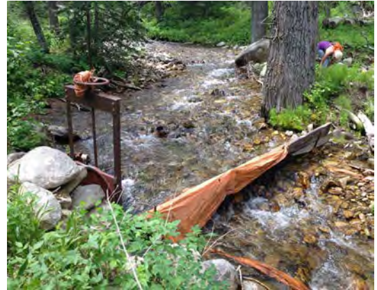
Replacement or maintenance of irrigation structures are common 310 projects.
