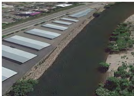
Bank stabilization projects longer than 300 feet will require stream mitigation under the Montana Stream Mitigation Procedures. Hard stabilization using riprap typically requires much more mitigation than bioengineering techniques.
