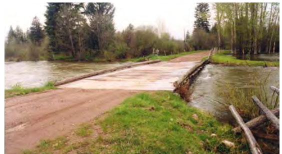
Stream crossings on shallow channels with broad floodplains must rise to meet the bridge, or the bridge will end up being too low, like this one.
