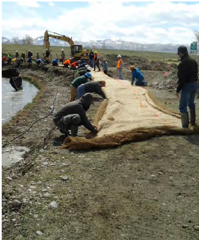
Fascines and brush layering can provide a foundation for less erosive environments.
