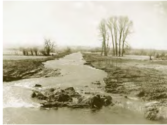
Channelization of streams frequently results in incised channels in disconnected floodplains. Big Spring Creek near Lewistown was channelized at the turn of the century.
