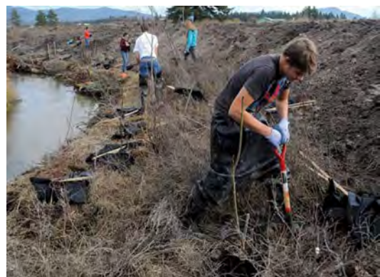
Willow stakes can be planted through fabric or into soils or sod.
