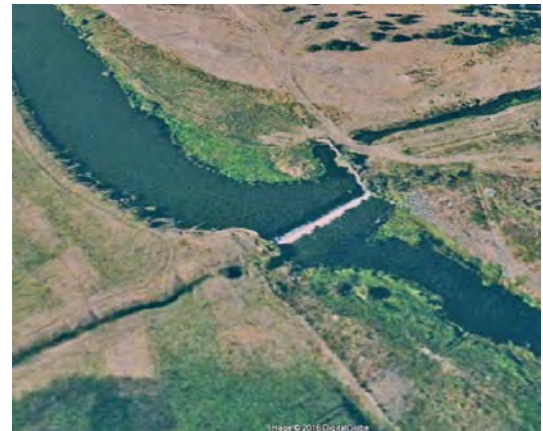
Irrigation dam prior to retrofit with engineered riffle bypass.
