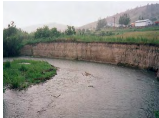
Eroding terrace before restoration on Rosgen C3 channel type.
