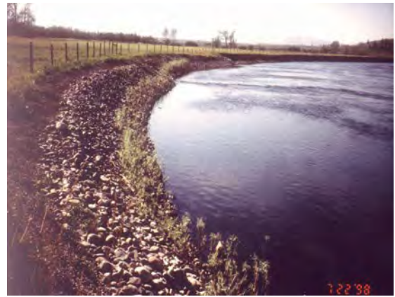
A bendway weir has a gradually sloping profile which shifts the main channel of the river to the outside of the structure. Peak flows continue to use the channel cross section above the weir elevation.
