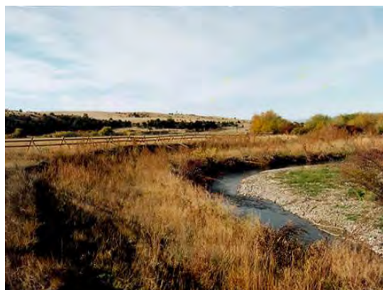
Terrace with brush layer toe and geotextile fabric bankfull bench. This project failed after three years and returned to a similar condition as pre-construction.
