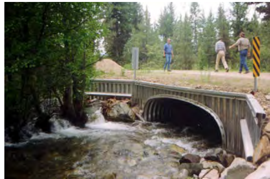
Bottomless arch or box pipes (shown here) promote fish passage and create less backwater than round pipes of the same size, but can be susceptible to scour.
