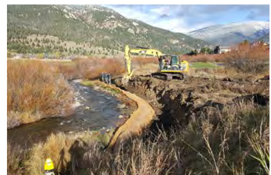
Installation of soil lifts requires excavating the streambank 10 or more feet.
