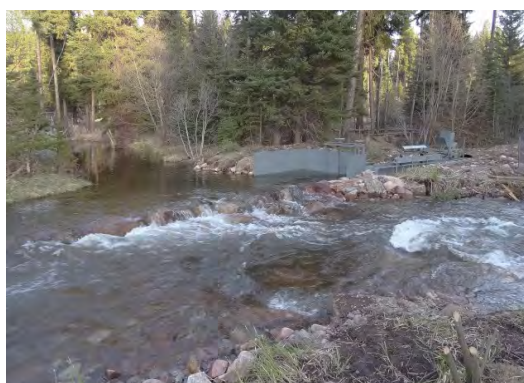
View of the diversion weir, engineered riffle, new radial headgate and flat panel fish screen.
