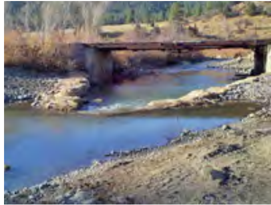
This crossvane weir is designed to control width-to-depth ratio alignment at a bridge cross section. Caution: sediment transport can be reduced causing channel instability in high bedload rivers.
