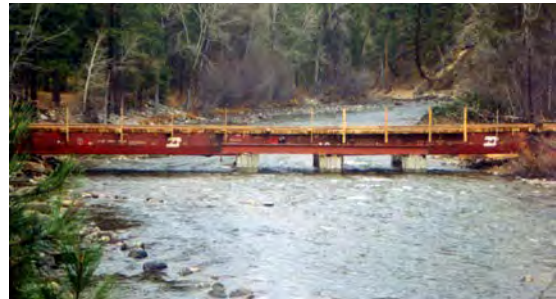
Railcar bridges are popular and fairly solid, but often are not installed properly. This one is set low relative to bankfull, but it is a temporary installation.
