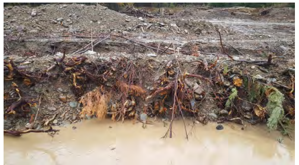
Ratio of brush and alluvium is dictated by local erosive forces.
