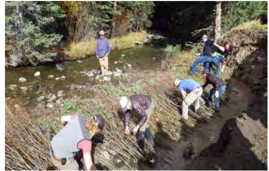
Base of willow cuttings should touch groundwater where possible.
