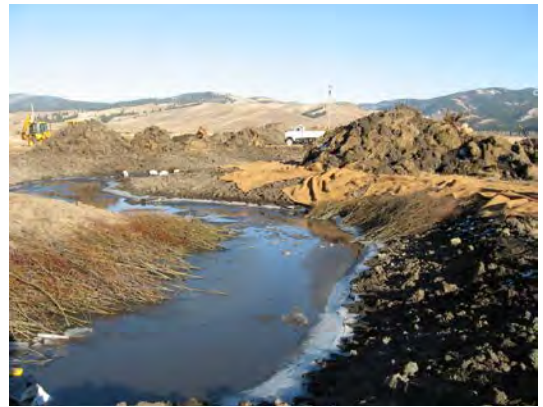
Soaking willows prior to planting is important to establishment. After two weeks of soaking fragile roots will emerge and may be damaged during planting.
