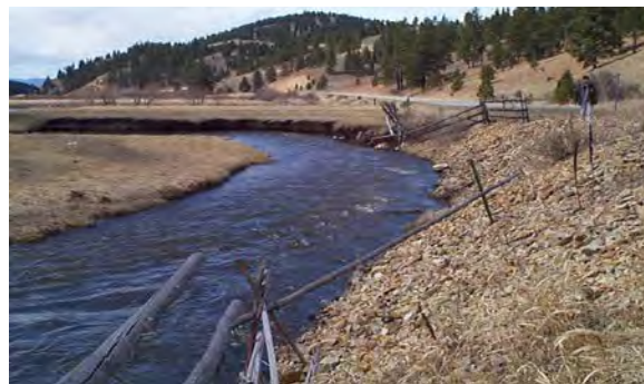
A well designed rip-rap job has 2:1 slopes and does not encroach on the river. This bank may have been stabilized using geotextile and vegetative methods with equal success. Note that Erosion has moved downstream below this rip-rapped bank.
