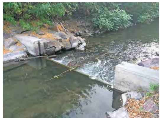
Rectangular weirs can be used to estimate flow if pooling of water behind structure is acceptable.
