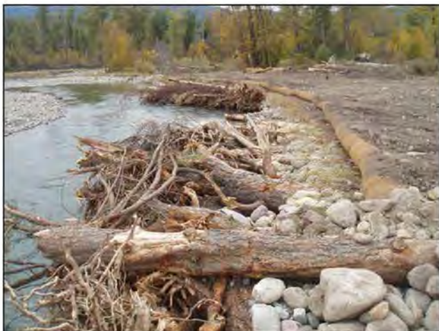
Example of a constructed large wood structure type 1
