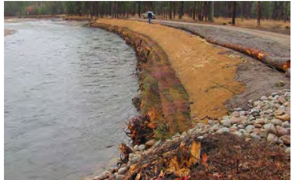
Encapsulated soil lifts with LWD toe and willow cuttings.
