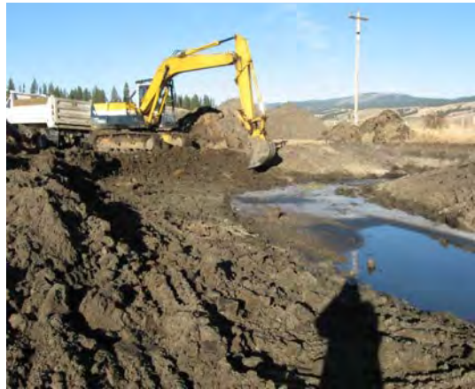
Construction should seek to minimize the amount of flowing water through the site.
