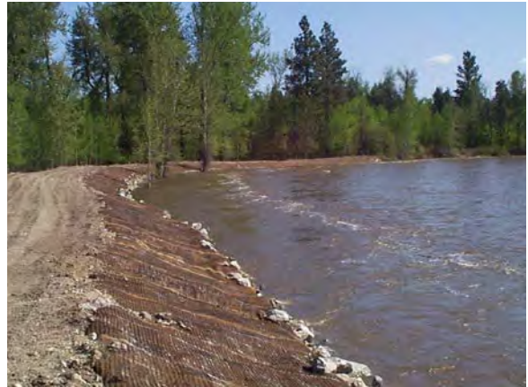
This dike was stabilized to protect downstream development from flooding, although the landowner with the dike did not particularly want to constrain the river.
