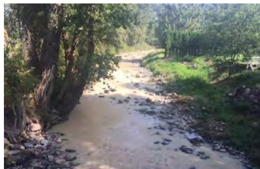
Releases of sediment during instream construction can cause substantial water quality impacts.
