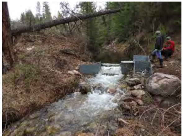
Fish screens can be installed in a stream, side channel, or ditch. Individual site constraints will dictate options that can be considered.
