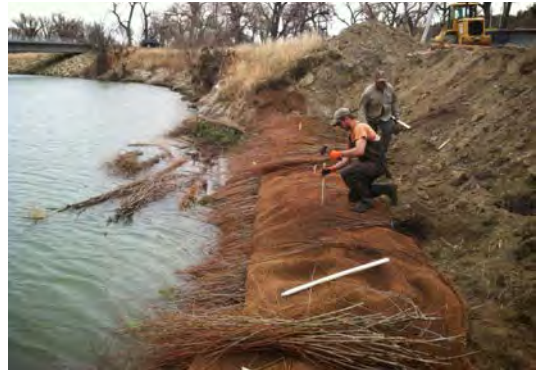
Brush layers have the best survival when placed near the water table or in moist soils. Irrigation may be required in droughty or coarse soils.
