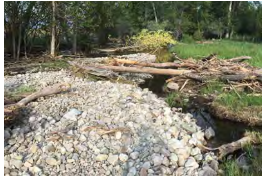
Aggrading (filling) channel reaches can be indicative of streams out of balance. This channel has completely filled with gravel delivered from upstream reaches.
