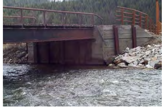
A well-constructed abutment has adequate wingwalls to support road fill.
