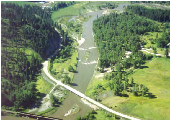
These large weirs eventually failed because they were built too high, and restricted sediment passage. Removal of these structures came at a high cost.
