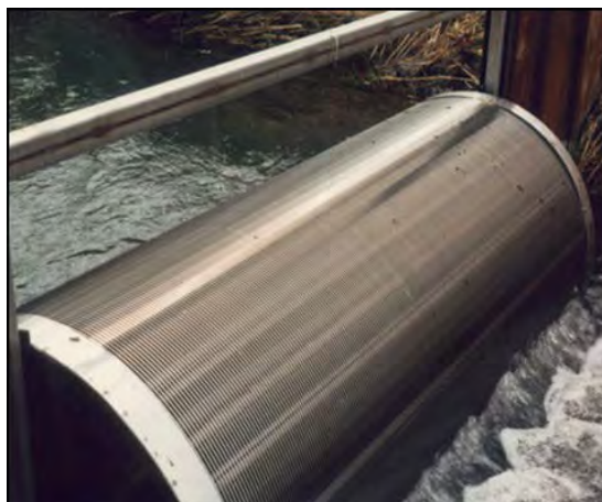
Inlets and outlets of ponds connected to perennial streams may require screening to prevent escapement of stocked fish, or capture of fish from the stream.
