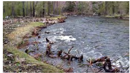
A completed soil lift with large woody debris toe emulates the natural range of bank roughness and stability.
