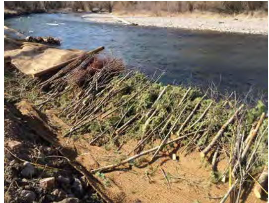
A mix of live and dead brush provides bank roughness and revegetation. A high density of stems (10-15 per foot) is common.
