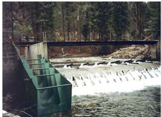
Denil fish ladders can function but are less desirable than constructed bypass channels. These are not recommended for bull trout passage.
