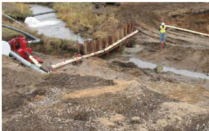
Pumping water around a construction site is generally feasible only on smaller projects and smaller flow rates.
