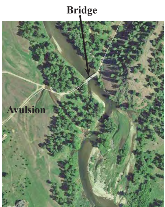
Bridge crossings and channel modifications require extensive hydraulic analysis for floodplain permitting.
