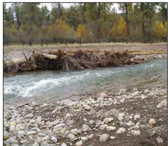
Example of a constructed large wood structure type 1
