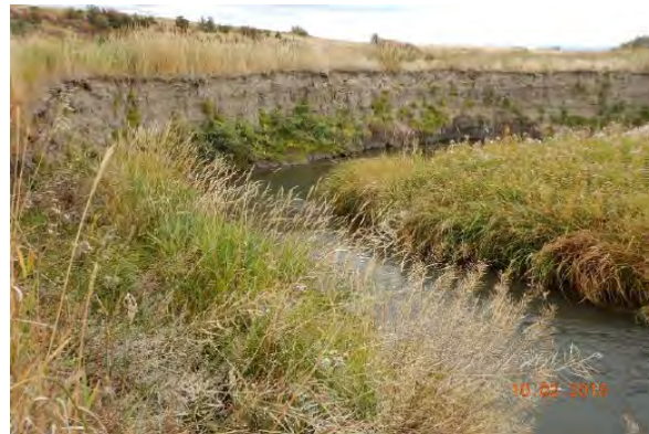
Before - An eroding bank (e.g., terrace or hillside) can sometimes be stabilized by construction of a bankfull bench. This may require channel reshaping to offset fill placed during construction of the bench.
