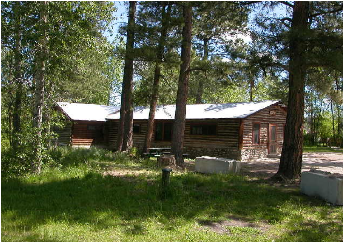
Structure at risk due to proximity of fire fuel, Stillwater County.
