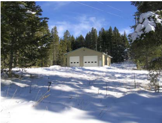
One of Three Georgetown Lake VFD Stations Photo Source: Russell Fox
