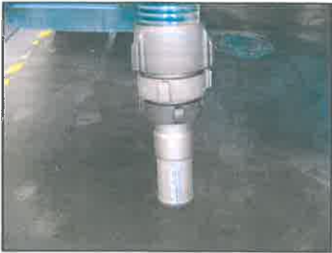
Figure 2. Foot valve attached to suction line with various adapters as needed to adjust for foot valve size.
