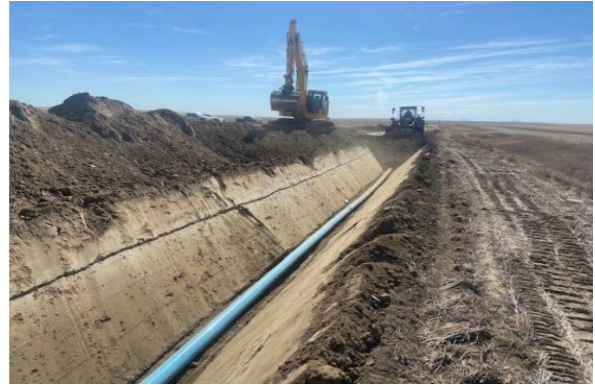
Pipeline construction north of Loma, 2022 -KLJ Engineering
