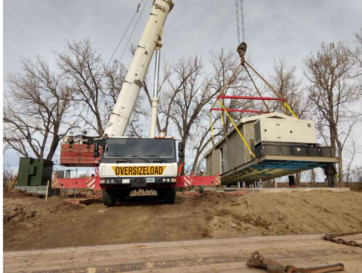
DRWA Sidney Circle Water Improvements, Nov 2018 – Photo by Interstate Engineering
