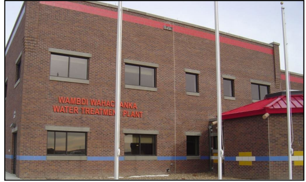
Wambdi Wahachanka Water Treatment Plant near Wolf Point
