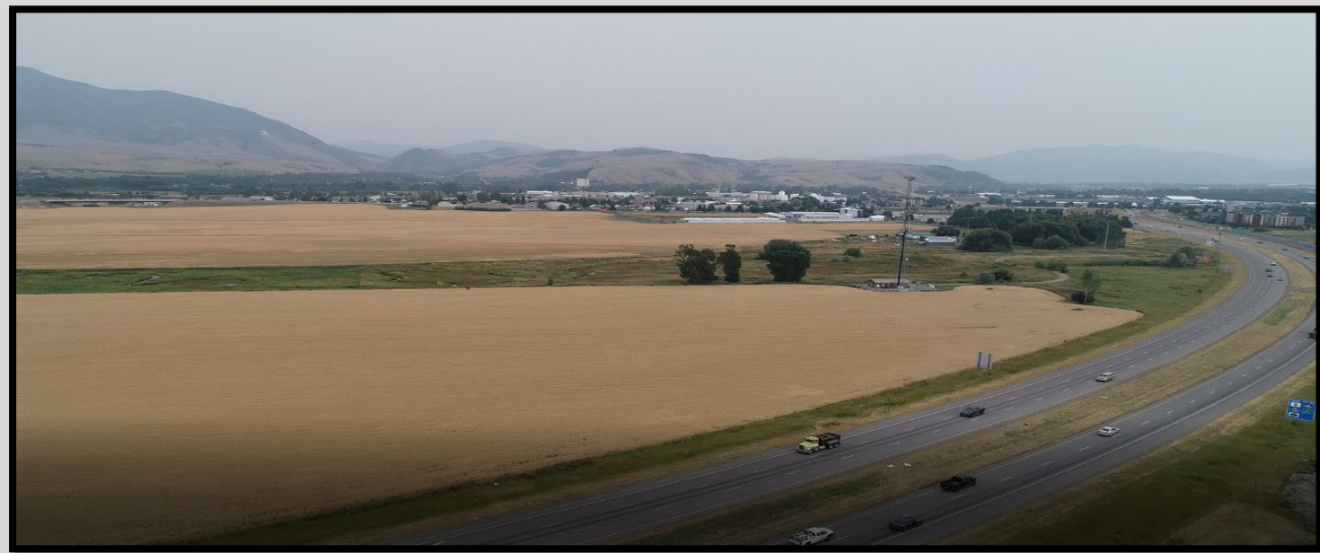
North Park – Bozeman – Infrastructure currently being installed.
