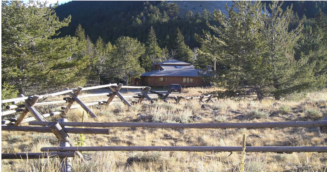
Figure 5-12. Picture of Home situated in the bottom of the West Fork of Rock Creek drainage.
