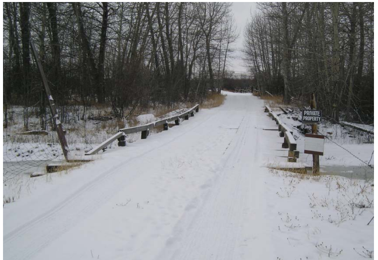
Figure 5-3. Picture of access across Rock Creek to Western Ranch Estates Subdivision
